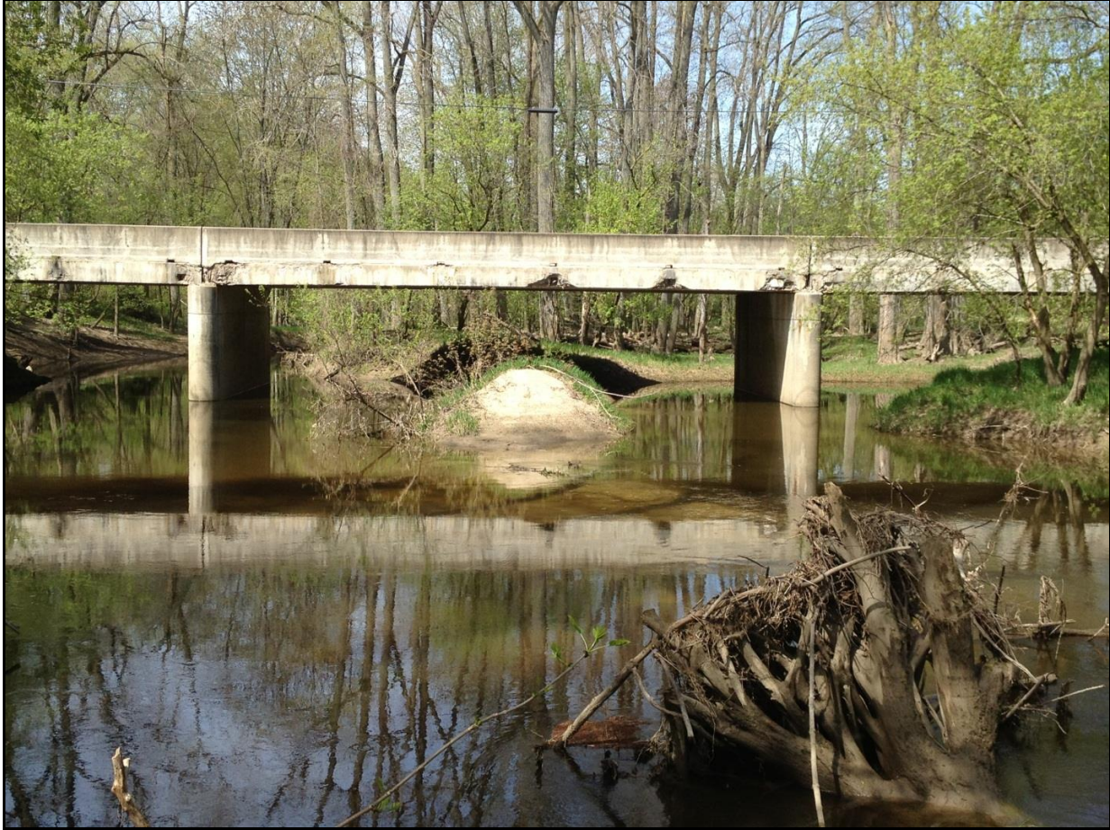
Figure 2.30 Belle River at Palms Road crossing (facing upstream)
