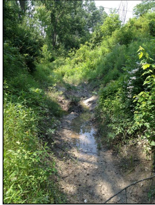
Figure 2.25 Example of channel downcutting in Schneider-China Drain (China Twp.)
