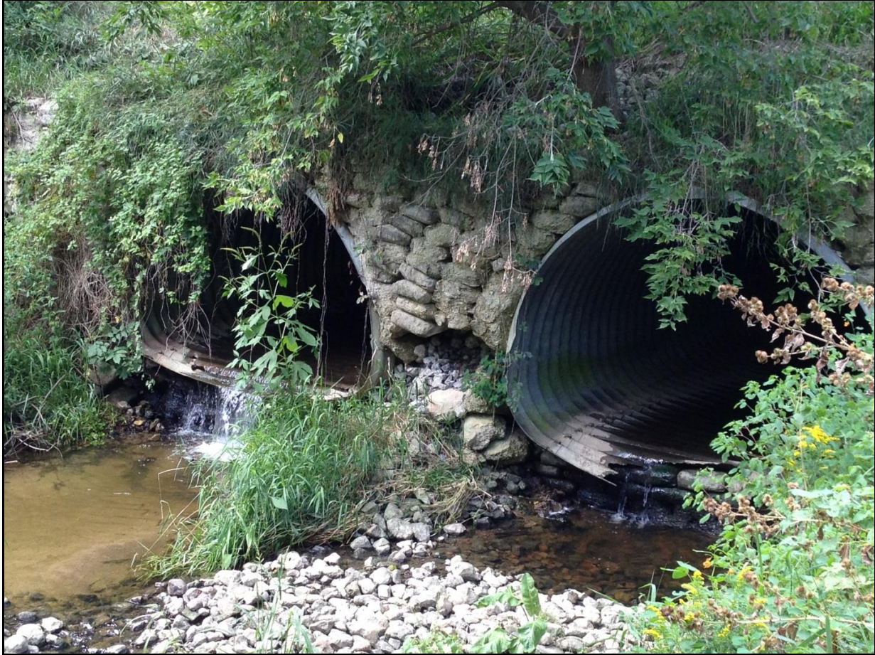
Figure 2.29 Jerome Creek at Church Road crossing (facing upstream)
