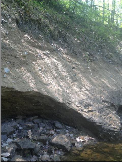
Figure 2.26 Hillslope failures on Belle River upstream of the Memphis gauge station
