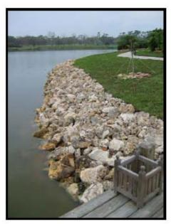
Figure 6.5 Example of Riprap Shoreline Stabilization Practice
