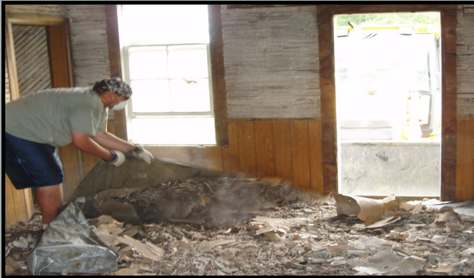
A worker removes plaster. The original plaster was badly damaged and could not be saved.
