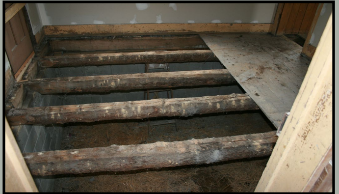
Some of the original chestnut floor boards needed to be replaced. Clues pointed to a kitchen fire.
