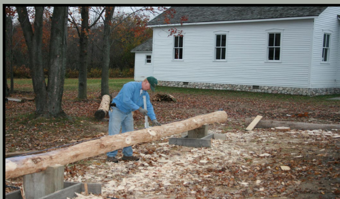
Park staff was trained to hand hew the logs for the cabin. This included using a broad axe and an adze.
