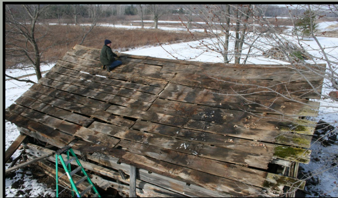
Staff works to remove roof boards. Most of the boards were salvaged and repaired.
