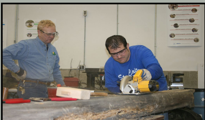
Some cabin logs needed some repair. Staff used a special epoxy to fill the rotted areas.
