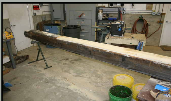
This log had a rotted top but was salvageable. It was repaired using a cap that was reshaped to match.
