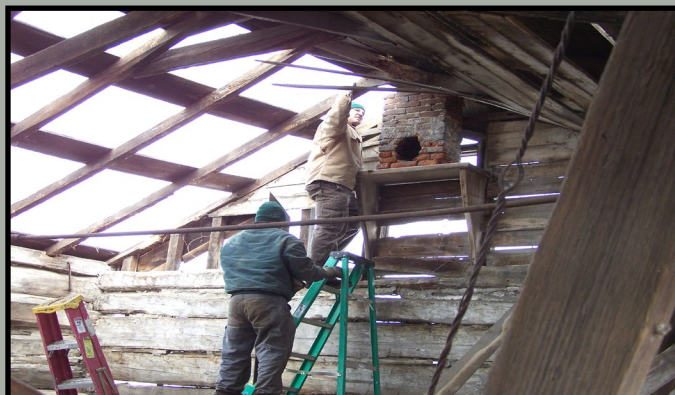
Staff carefully removes the original brick chimney. The unique chimney sat on a wood platform.
