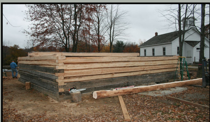
The cabin being reassembled, using original and replacement logs.
