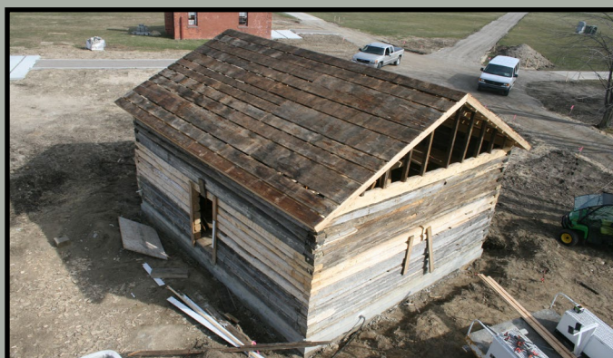
The roof boards after being reinstalled. These can be seen in the before photo at the top of the page.
