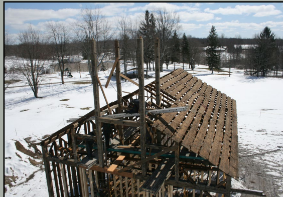
The original belfry was removed in the 1950s. By using original markings and photos, the belfry was re-created.
