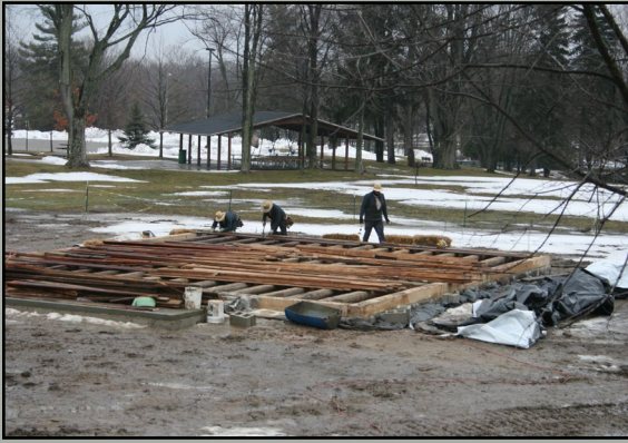
Original floor joists being reinstalled on a new foundation
