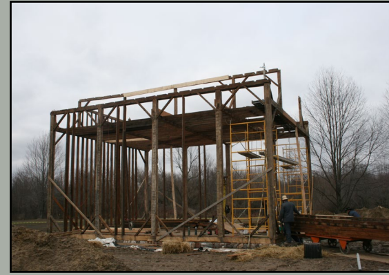
Summer beams and girts are reinstalled. These are the horizontal posts that connect to the wall posts
