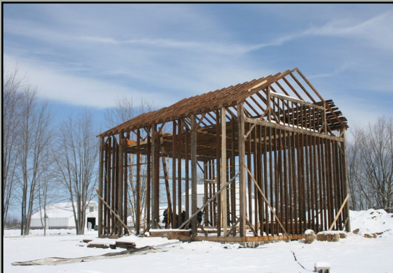
Wall studs and rafters are installed. Over 90% of this material is original.
