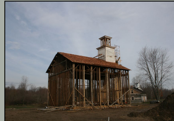
Belfry taking shape and the Cedar shingles are installed.
