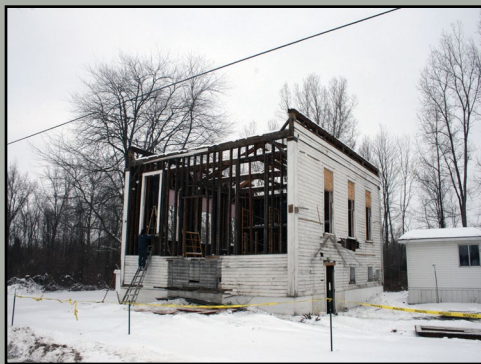
9 Roof trusses and front siding removed 1/14/2011.
