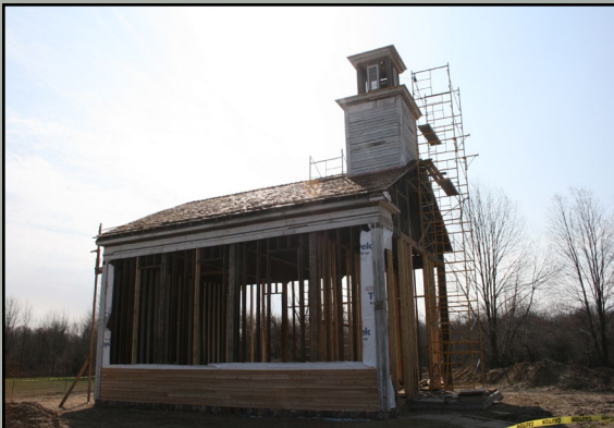
Siding being installed.
