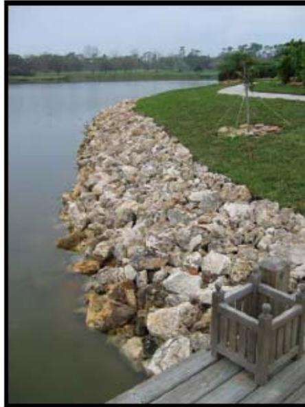
**Figure 6.5 Example of Riprap Shoreline Stabilization Practice**
