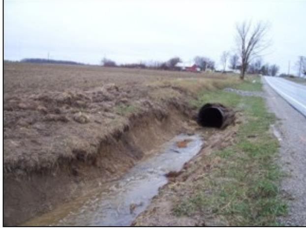
**Figure 3.3 Un-vegetated Drainage Ditch**
